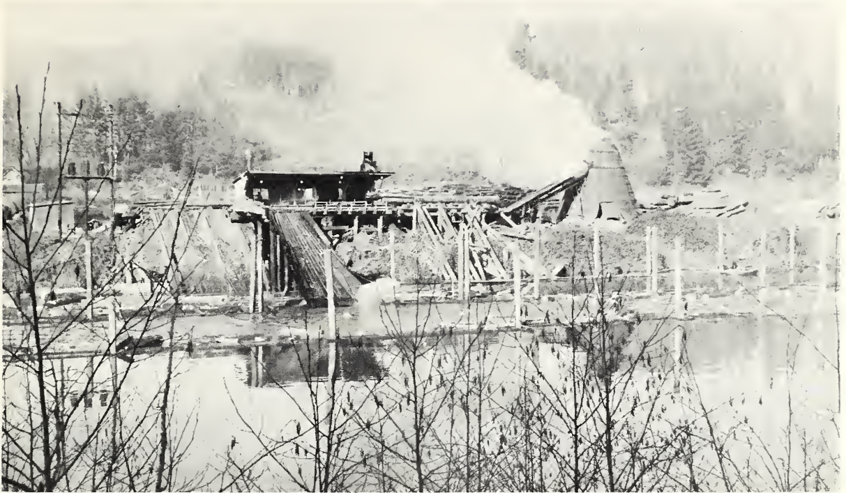
Photo 21.--Peeler blocks are transported from the cut-off saw to the plywood plant by the current of the Siuslaw River. Poppino photo NO. 1
